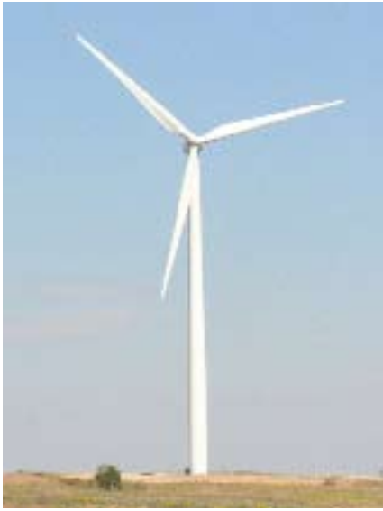
A wind turbine at the Weatherford wind farm generates electricity for western Oklahoma. (photo by Everett Brazil III.)
